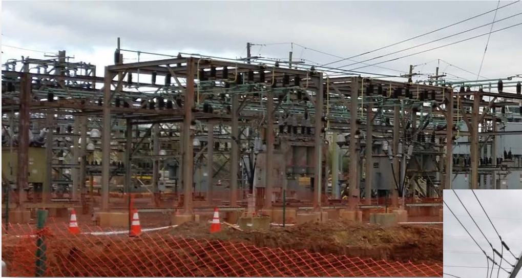
Sewaren Switching Station – Before
